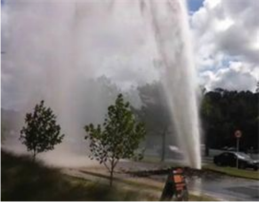
Failed watermain and associated flooding, Albany.
